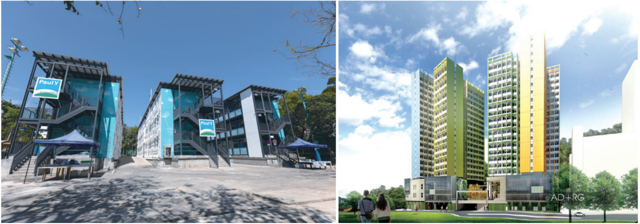
(左) 於西貢戶外康樂中心內之臨時隔離營 / (右) 香港大學黃竹坑學生宿舍 Left: Temporary quarantine facilities (TQF) built using MiC by Paul Y Engineering; Right: HKU's Student Residence at Wong Chuk Hang (Copyright by AD+RG)
