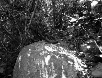
Figure 15: One of the iron rings found along the steps leading to the gun emplacements of D'Aguilar Battery
