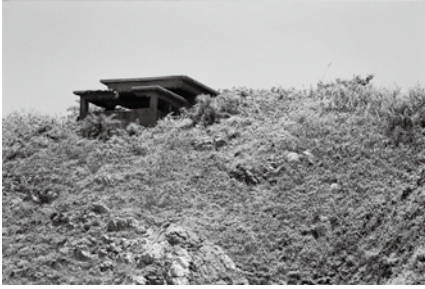
Figure 10: Battery Observation Post, Bokhara Battery, 2003
