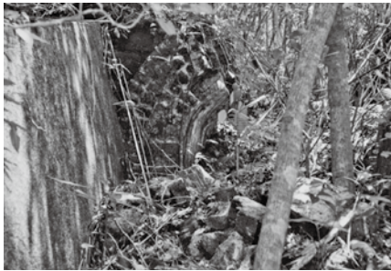
Figure 8: Demolished tunnel entrance PB 123 (Author's photo taken 1995)
