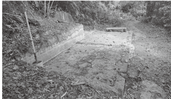
Figure 5: The remains of concrete walls mark the original layout of the two-room shelter. The path to the rear connects to Po Lam Road South (photo by author in 2019).
