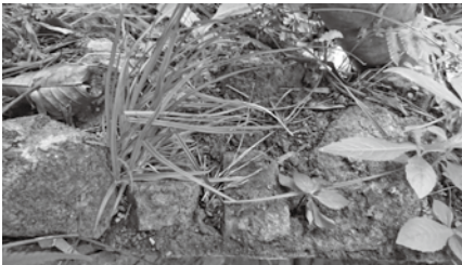
Figure 7: The walls of the small room in the back were made of big rocks that provided less protection than concrete, which probably had to be rationed for more important parts of the structure (photo by author in 2019).
