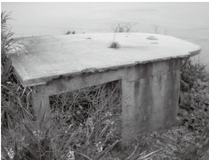
Figure 11: The right searchlight position below Bokhara Battery, 2006
