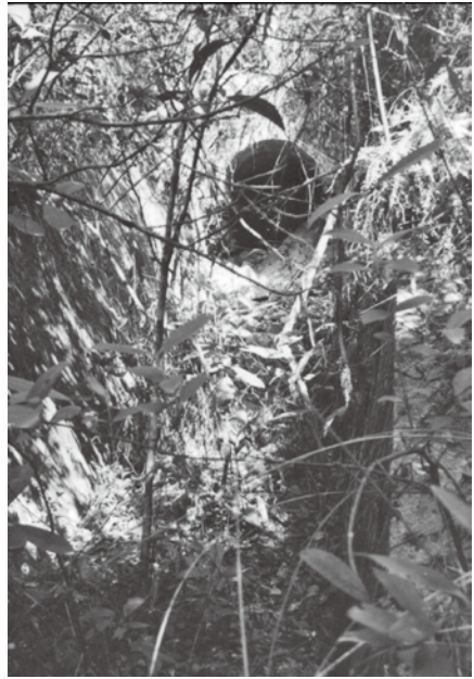
Figure 6: Entrance to PB 314 as found (Author's photo taken 1995)
