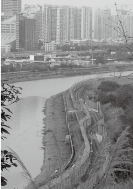
Figure 5. Road along the Border
