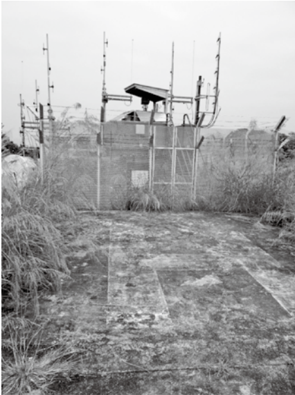
Figure 19. Helipad at Wu Shek Kok
