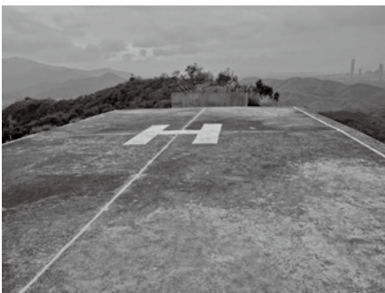
Figure 20. Helipad at Crest Hill
