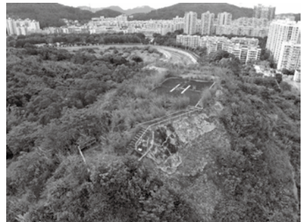
Figure 17. Helipad at Pak Fu Shan Police Post
