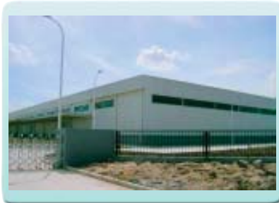
▲ UPS new distribution facility in Waigaoqiao Free Trade Zone
