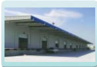
▲ One new warehouse in Waigaoqiao International Logistics Park
