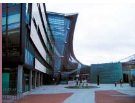
Entrance to the technology centre of the complex
