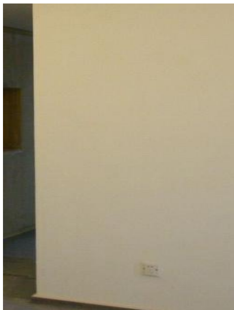
Picture 8a Switch at Low Level
