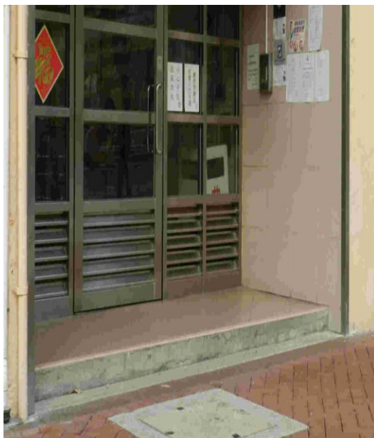
Picture 6a No Ramp at Entrance
