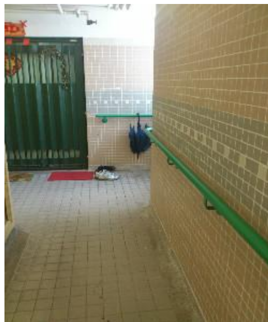
Picture 9b Handrails along Corridor
