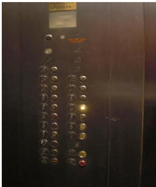
Picture 3 Too Small Lift Buttons
