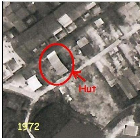
Figure 20 Enlarge aerial photograph in 1972 showing the hut Year of 1980, 1996, 2003
