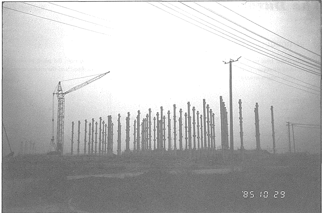
Prefabricated Factory under Construction in Minhang Development Zone
