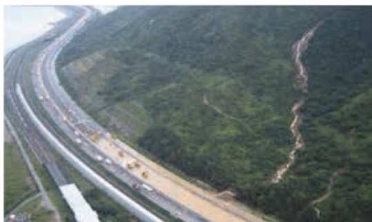
Figure 3 – Trunk Road to the HK International Airport was Cut Off by Debris Flows and Flooding in June 2008
