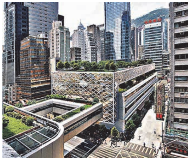
Fig. 2 The Central Oasis Project, adaptive reuse of the Central Market for shopping and public recreation and entertainment. (Source: AGC Design Limited)
