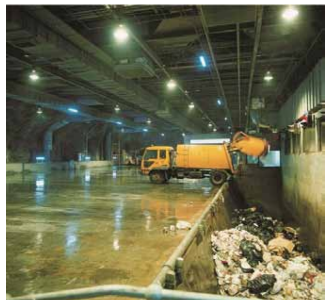
(Island West Refuse Transfer Station Inside Cavern)
