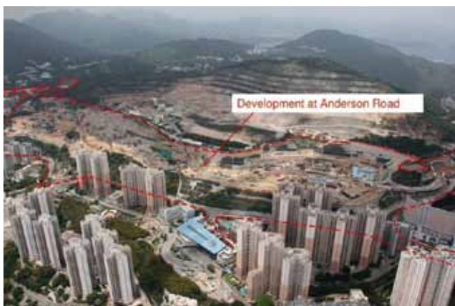
(Site of Development at Anderson Road Project)
