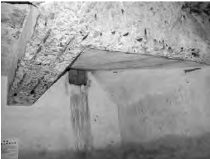
Figure 26: Roof of a kitchen in the “Strand Palace Hotel”.
