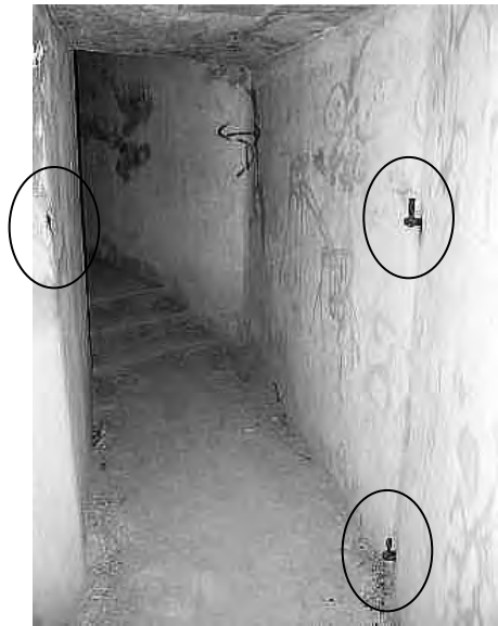
Figure 23: the Gate to PB400.
