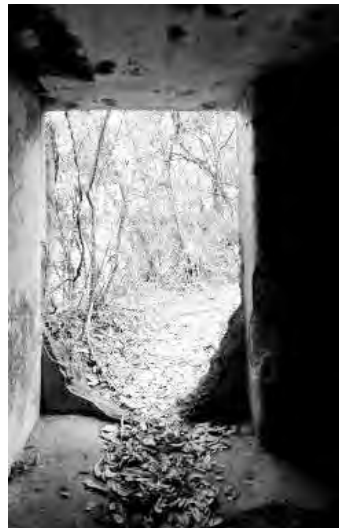
Figure 21: The emergency exit (?) from the inside.
