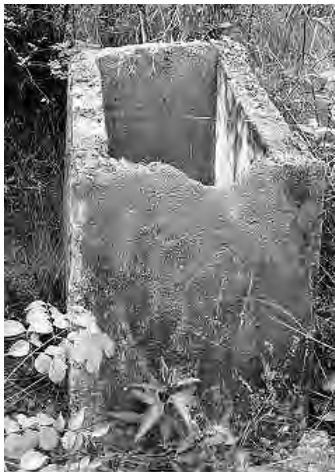
Figure 19: Ventilation shaft near Structures X and Y.
