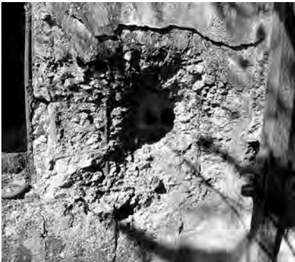
Fig 5: Penetrating hit mark on exterior of PB20's searchlight shelter on Hong Kong Island.
