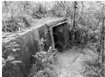
Figure 22: The emergency exit (?) on the outside.
