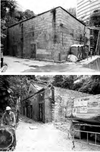
Figure 3: The two explosives magazines before they were adapted as part of the cultural facilities of Asia Society Hong Kong Center. (Photo credit: Lee Ho Yin)
