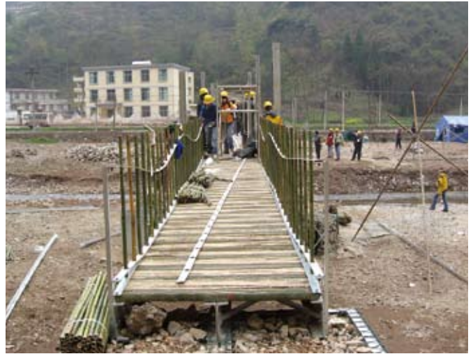
Bamboo railings were installed
