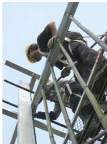
Works at high level
