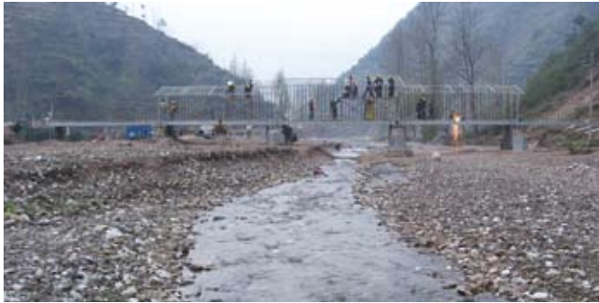
Bridge nearing completion
