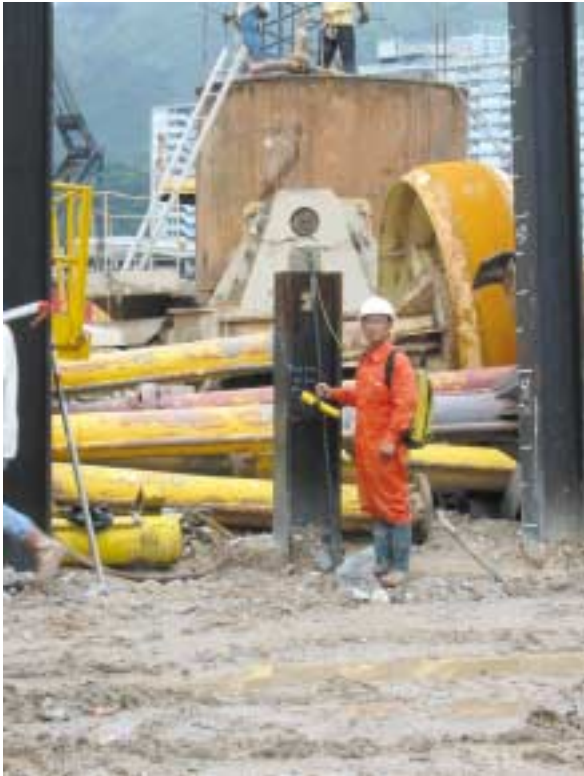
Figure 2 GPS antenna on top of the pile
