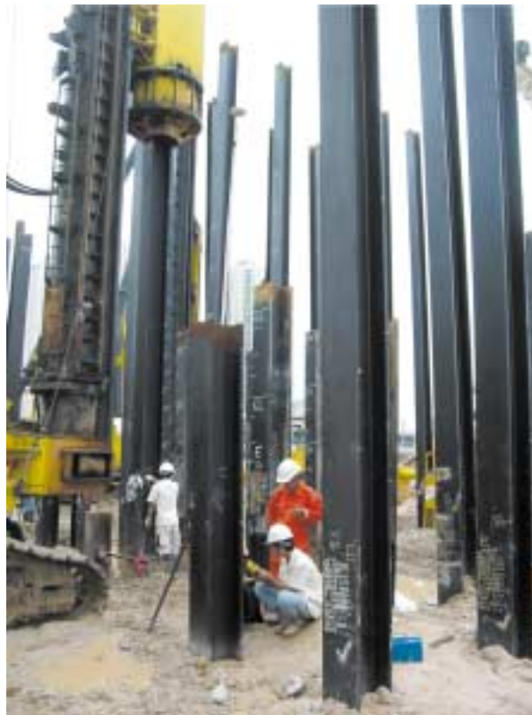
Figure 1 Construction site with lots of piles
