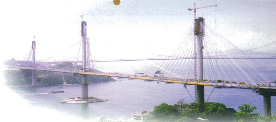
Ting Kau Bridge at the Construction Completion Stage
